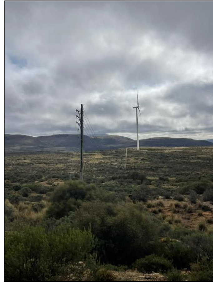
2. Monopole infrastructure in place
