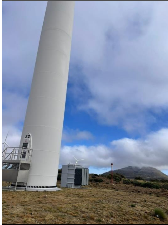
1. Image representative of conditions around the base of towers
